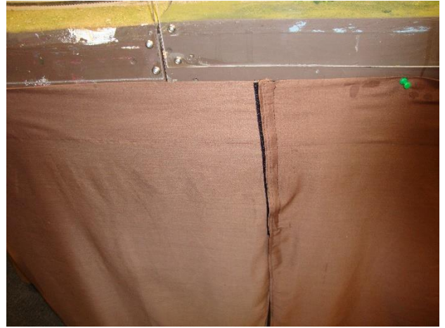
Figure 15 – Connected and stretched skirt sections
