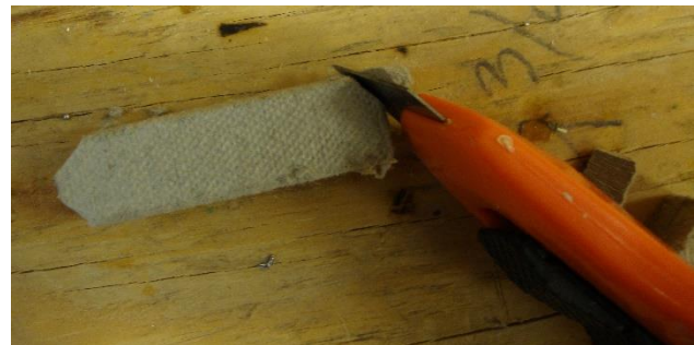
Figure 10 – Trimming plug
