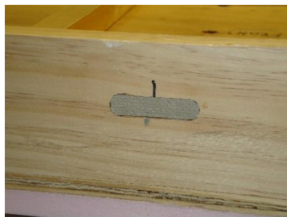
Figure 12 - Plug glued into cavity
